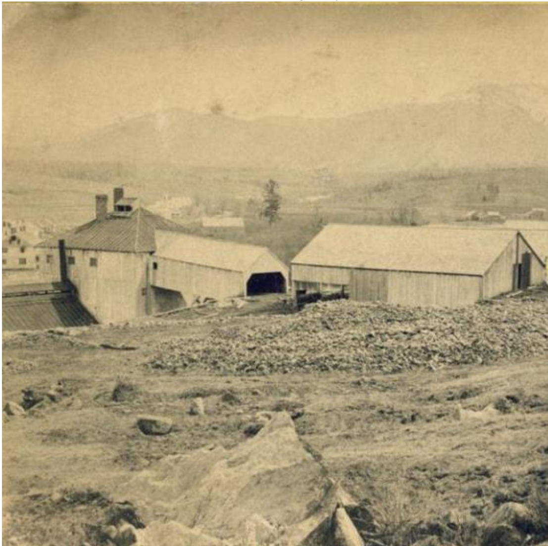
The furnace was enclosed within the building with the gambrel roof.
