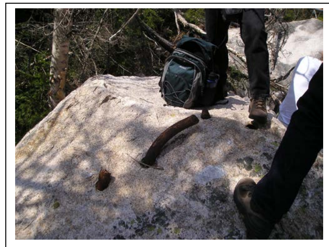
Fig 2. Forensic geology-the twisted and broken steel rods, epoxied into drill holes, confirm the blocks were part of the Old Man..
