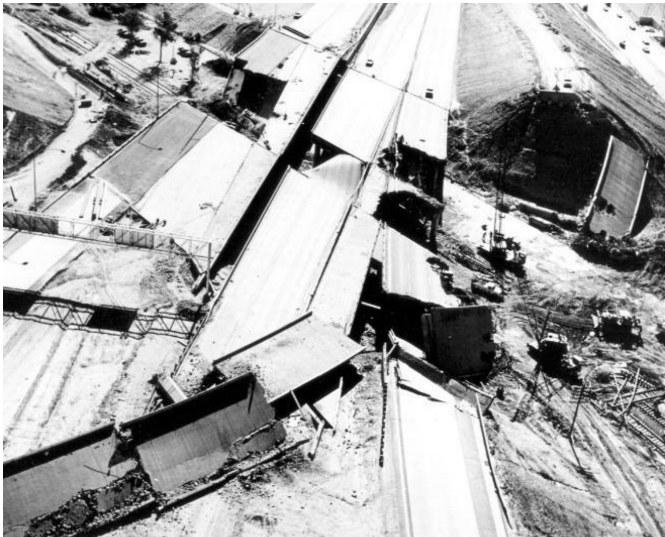
Oblique aerial view of collapsed highway overpasses and bridges at the interchange of the Foothill and Golden State Freeways after the San Fernando earthquake in February 1971. The principal highway link between northern and southern California was temporarily cut and traffic had to be re-routed for several months. (Credit: R. E. Wallace, USGS. Public domain.)
