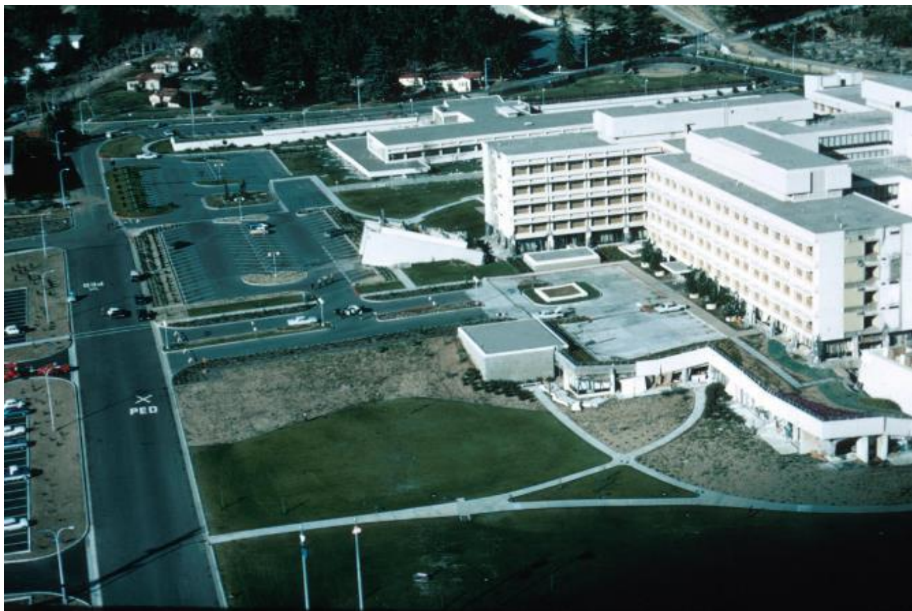
Two fallen structurally separated stair towers and the collapsed basement at Olive View Hospital after the San Fernando earthquake in February 1971. View is north. (Credit: USGS. Public domain.)
