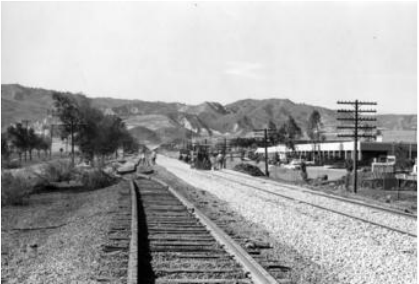
Photo showing railroad track damage following the San Fernando Earthquake on February 9, 1971. (Credit: USGS. Public domain.)
