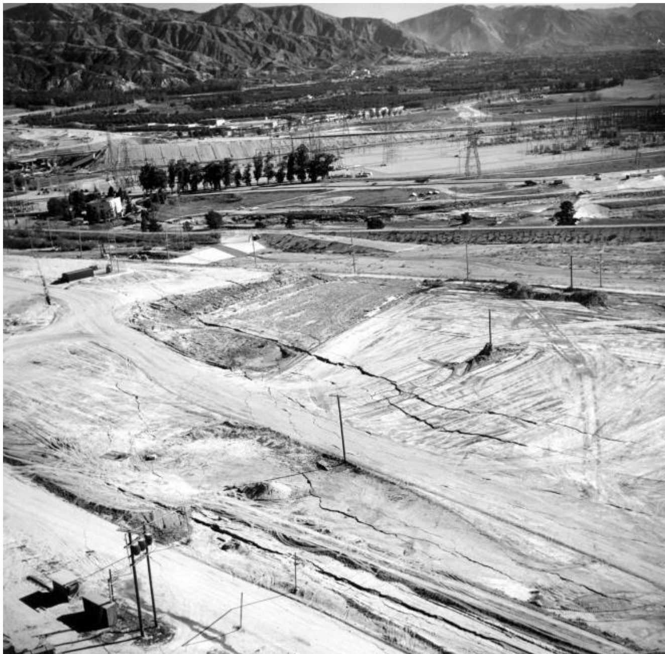
North-Trending fracture pattern near the Sylmar Converter Station above the upon Van Norman Dam. The fracture was due to a landslide and the dam's setting in extensive fill material. Photo taken from a view looking northeast on Feb 10, 1971. (Credit: USGS. Public domain.)
