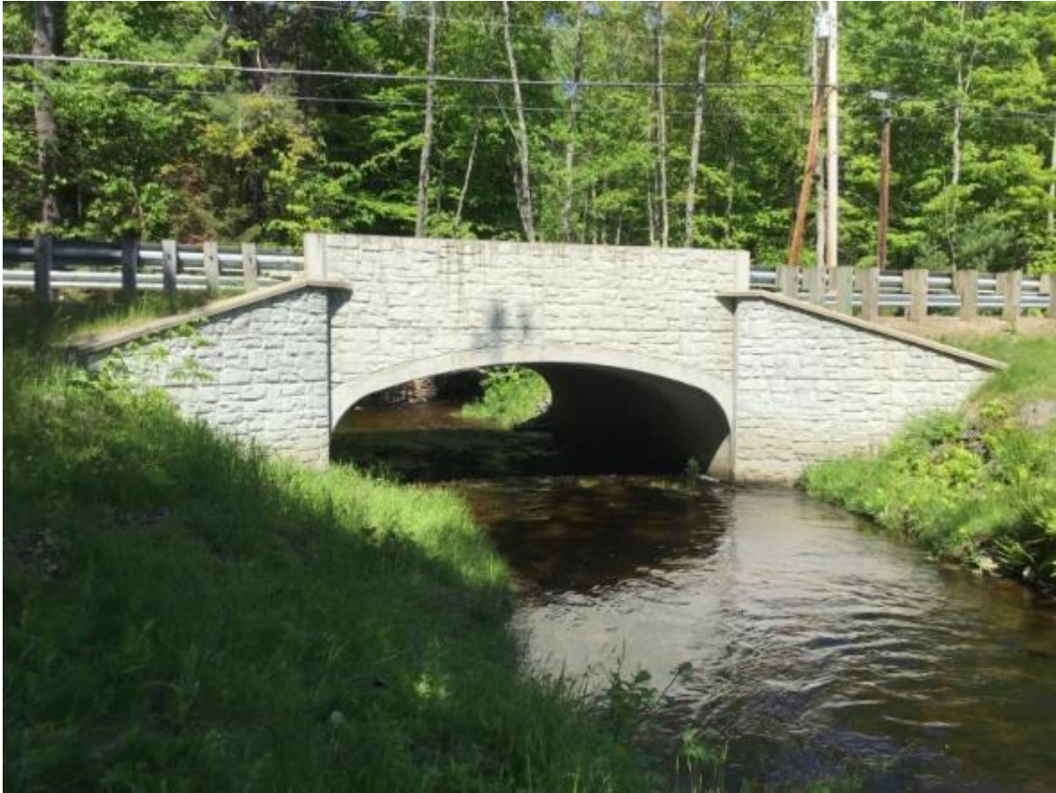
Local culvert under evaluation. Submitted by Shane Csiki.
