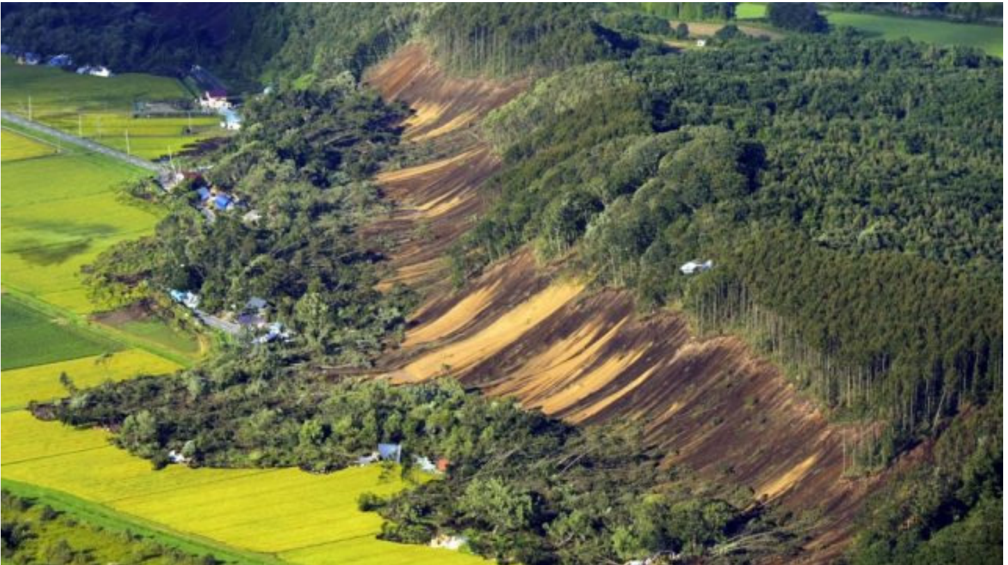
The ridge failure landslides from the 6th September 2018 Hokkaido earthquake. Image via SCMP .
