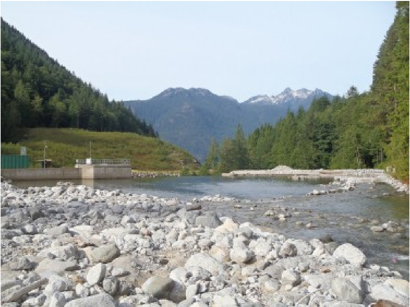
A 22-megawatt small hydroelectric project on Stokke Creek in British Columbia, Canada. Rylee Murray
