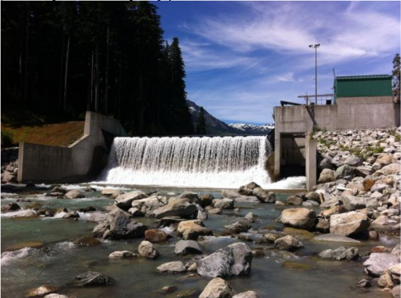
A small hydropower dam on Rutherford Creek in British Columbia, Canada. This dam produces 49 megawatts of power. Rylee Murray
